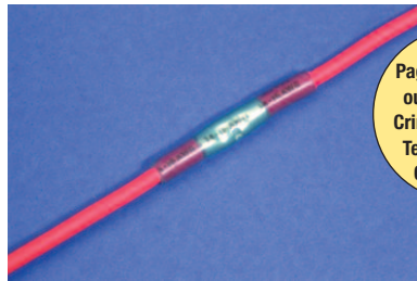
5. Completed Waterproof Connection
